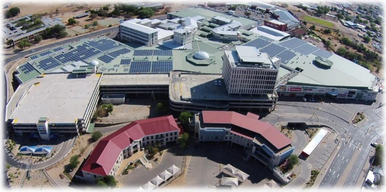
Maerua Mall, Windhoek, Namibia: 1 040 kWp Grid tied system, installed by NEC
