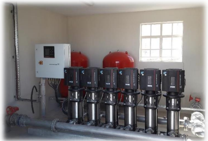
Pump Installation at Omuthiya Police Station & Grundfos Hydro 2000 pump
