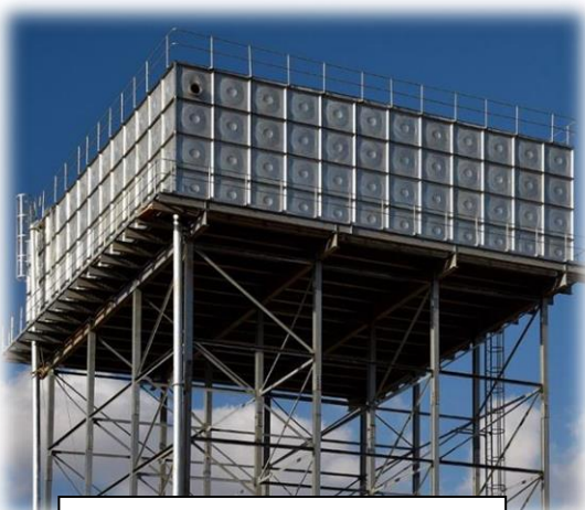
Large-scale elevated water Tank
