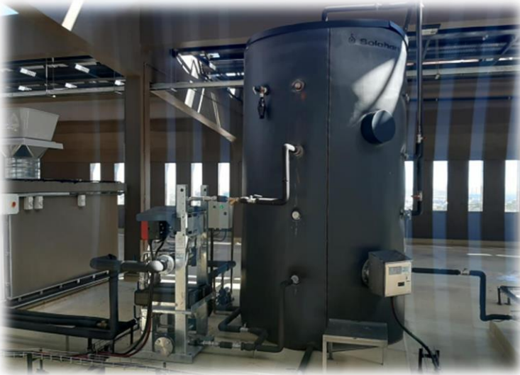
Ministry of Home Affairs & Security – Head Office in Windhoek 2 X 5000 Storage tanks with solar pump skid & solar delivery skid & 28 x LCS collectors
