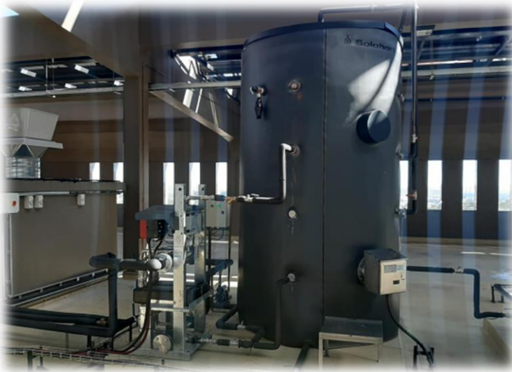
Ministry of Home Affairs & Security – Head Office in Windhoek 2 X 5000 Storage tanks with solar pump skid & solar delivery skid & 28 x LCS collectors
