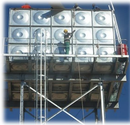
Elevated Water tank installation at Bethanie, Southern Namibia
