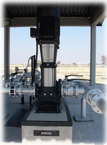
Pump Installation at Omuthiya Police Station & Grundfos Hydro 2000 pump
