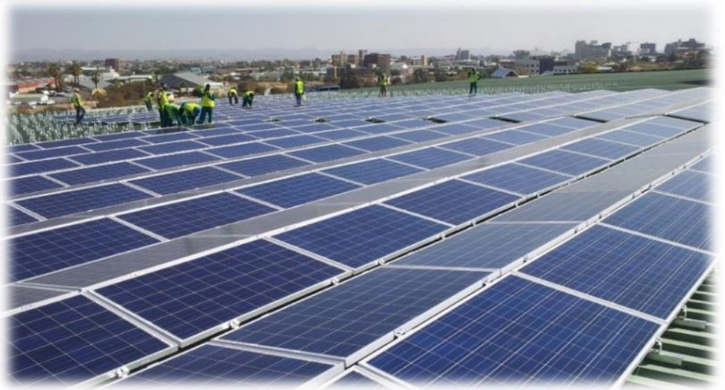
Maerua Mall, Windhoek, Namibia: 1 040 kWp Grid tied system, installed by NEC
