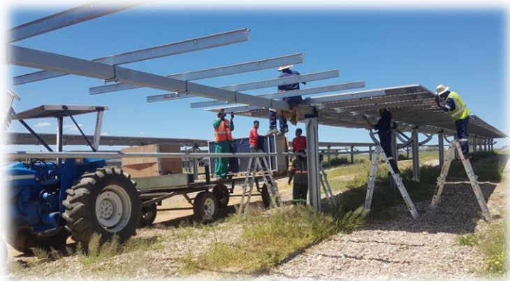
Namibia Poultry Industries Solar Farm completed 2022: Panel packing on modified trackers with reflective gravel underneath for bifacial effect of the panels increasing panel output by 5%.
