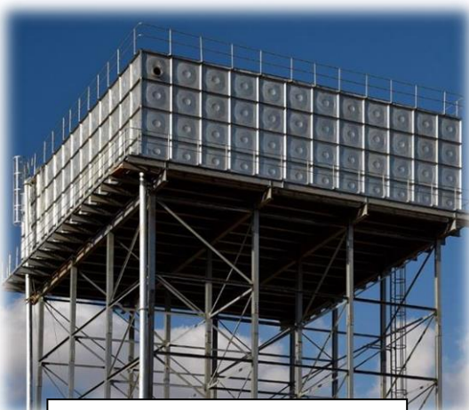
Large-scale elevated water Tank
